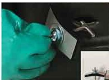
New Offset T Patches for holes & cracks near edge of tank
